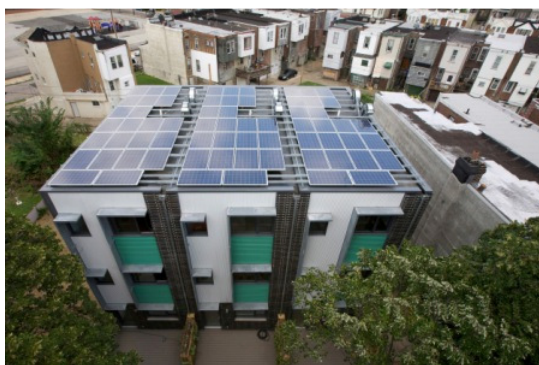
Belfield Homes (Philadelphia, USA). Photo: Sam Oberter Photography
