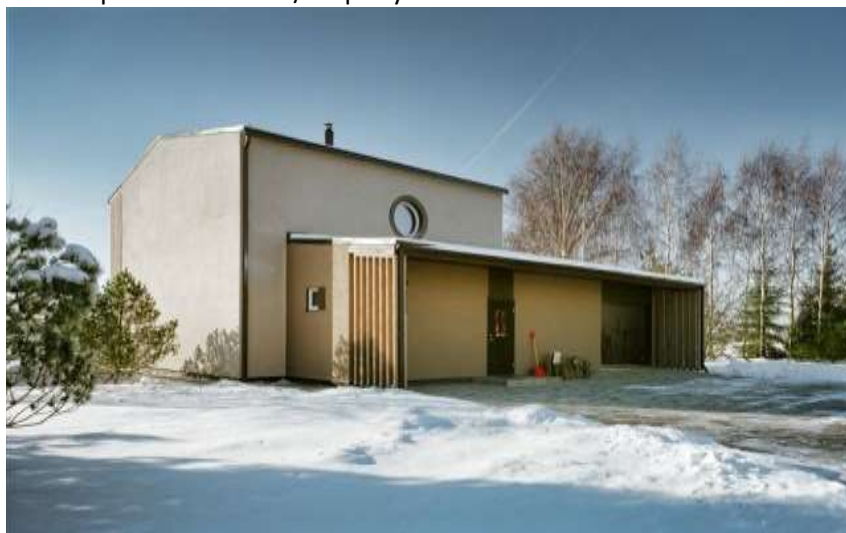
Figure 20. “Daugaviņas”, northern elevation. Source: Architect Ervins Krauklis
